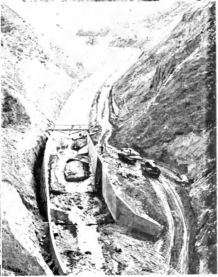
Top picture shows completed portion of flume, paralleling Grapevine Grade highway, for carrying creek waters past side area. Lower pictures show work on reinforced concrete lining of flume and the special spillway construction at its lower end.
